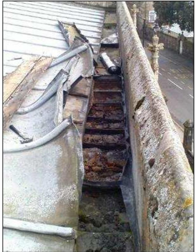
Our architect found that the boards supporting the gutters were rotten and needed urgent replacement.
