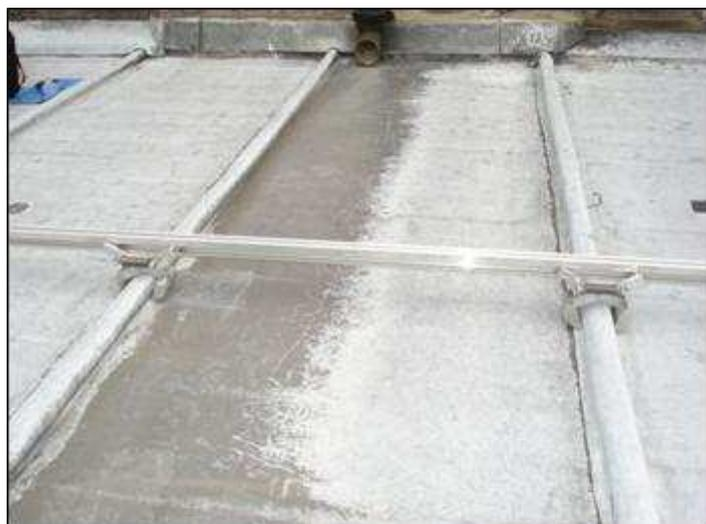
The 'Solstice' lead roll clamps in action on a tradition church roof.
