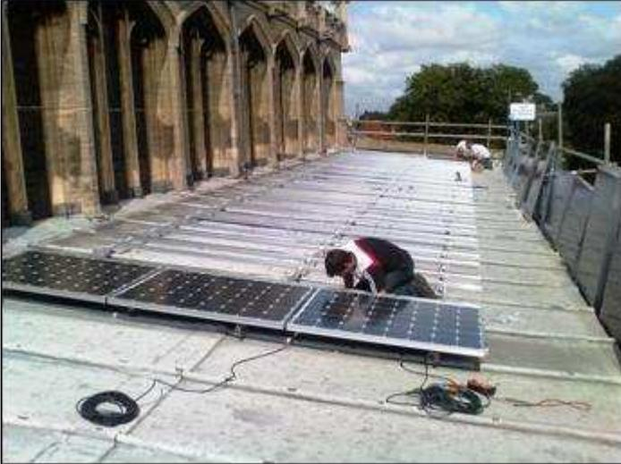
The panels are fitted to the framework and the cables are laid to carry the dc electricity generated by the panels to the inverters where it is converted to ac electricity ready for use in the church, or to be fed into the Grid.
